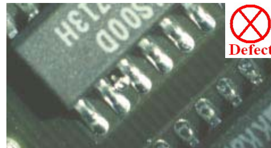
Defect Figure F2-3: Solder balls violate minimum electrical clearance Pin 脚间有锡球
